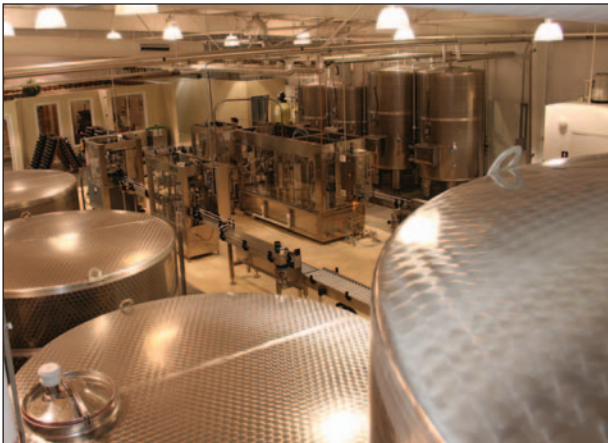
Figure 5. A winery needs to have tanks in several sizes to accommodate a variety of operations. (Photo courtesy of Prospero Equipment Corp.)
