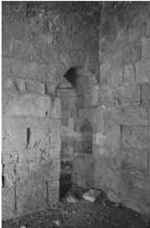
Fig. 12: Trapeza church passageway from central apse
