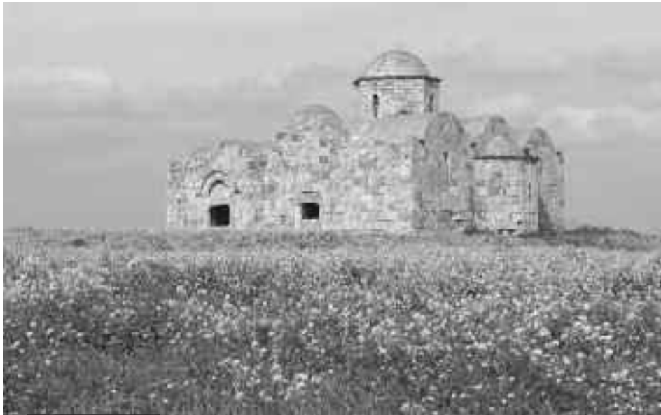
Fig. 2: The Trapeza church from the southeast
