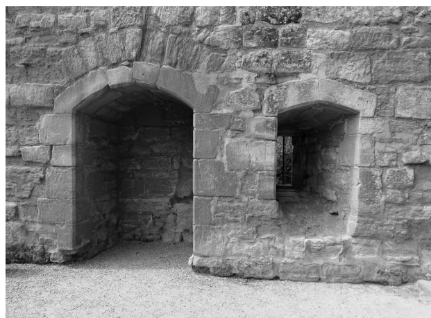
Fig. 3.28: Double latrine and window at northern end of western range with inconsistent chamfers. Photo by Penny Copeland.
