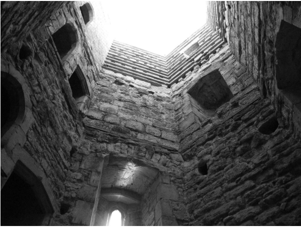
Fig. 3.36: Interior of south-west tower, with two lodgings and a dovecote above, partially restored. Photo by Penny Copeland.
