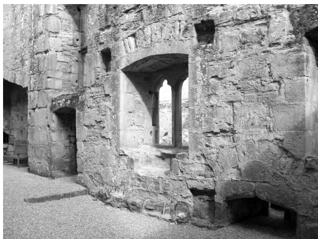
Fig. 3.26: Window to basement of service range excavated by Curzon, also showing the substantial mortices for wall partitions. Photo by Penny Copeland.
