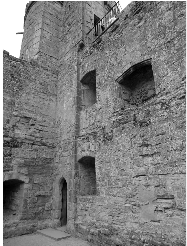
Fig. 3.30: Possible straight joint between north-west tower and north wall. Photo by Penny Copeland.
