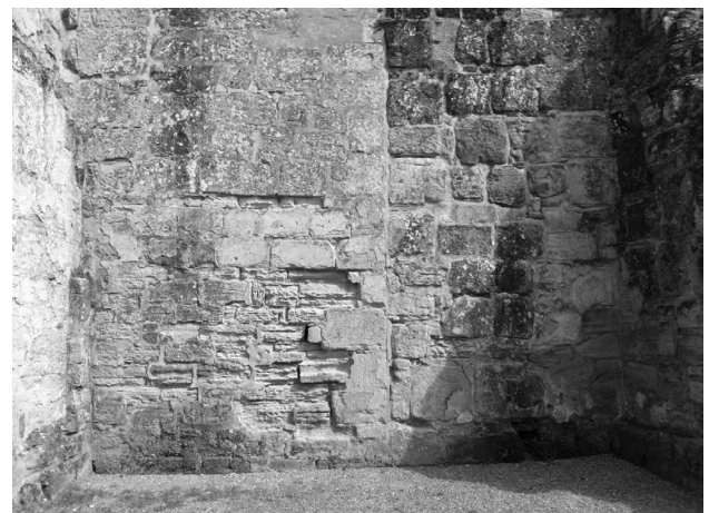
Fig. 3.16: West side of gatehouse showing the straight joint between the original and the southern sections. Photo by Matthew Johnson.
