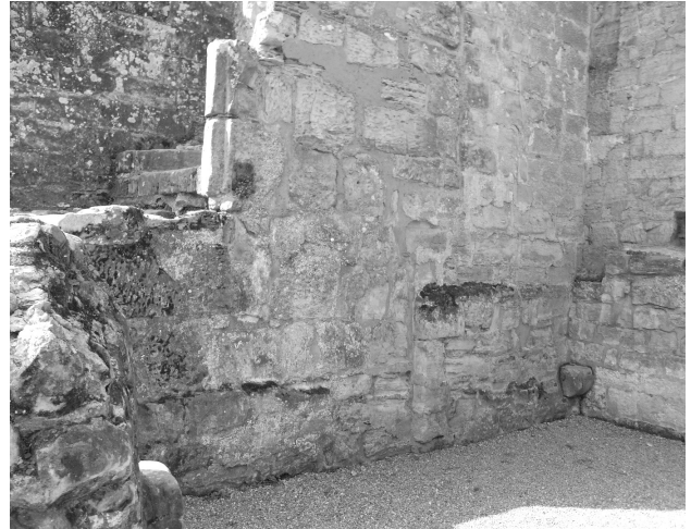
Fig. 3.18: Plinth to the east of the gatehouse showing a slight misalignment reused to support a beam. Photo by Penny Copeland.
