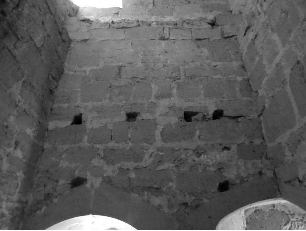
Fig. 3.11: Evidence for inserted floors, western ground floor room of gatehouse. Photo by Penny Copeland.
