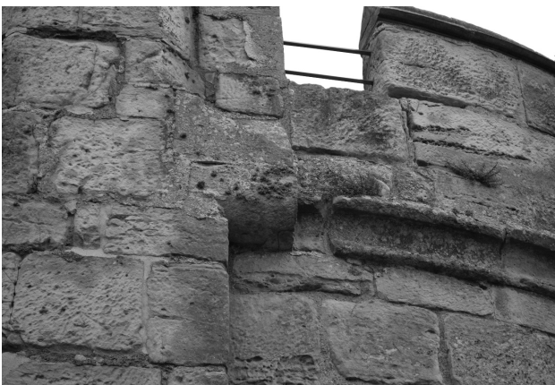
Fig. 3.29: Change from corbel to string course on the north-west tower. Photo by Penny Copeland.
