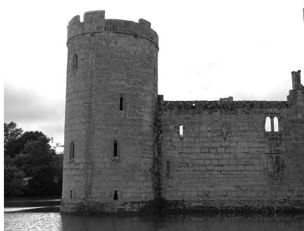
Fig. 3.31: Southern section of the east curtain wall showing different building seasons. Photo by Penny Copeland.
