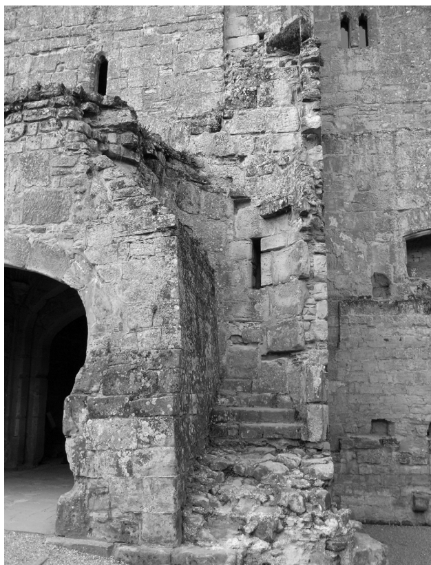
Fig. 3.14: Buttress against gatehouse, built up against stair to reach chamber. Photo by Penny Copeland.
