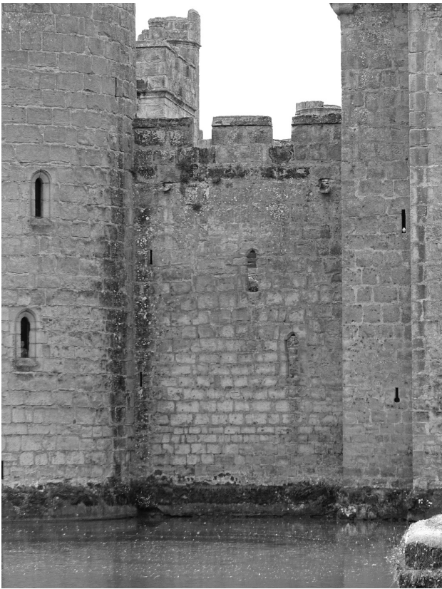
Fig. 3.20: Straight joint in external wall to east of gatehouse. Photo by Penny Copeland.
