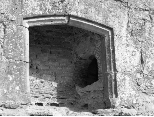
Fig. 3.24: Fireplace in main range that connects through to east tower recess. Photo by Penny Copeland.
