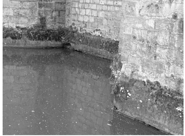
Fig. 3.13: Curzon's render to the plinth or 'apron'. Photo by Penny Copeland.
