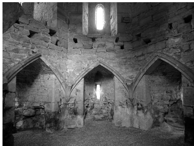
Fig. 3.35: Vaulted basement room of the south-east tower. Photo by Penny Copeland.
