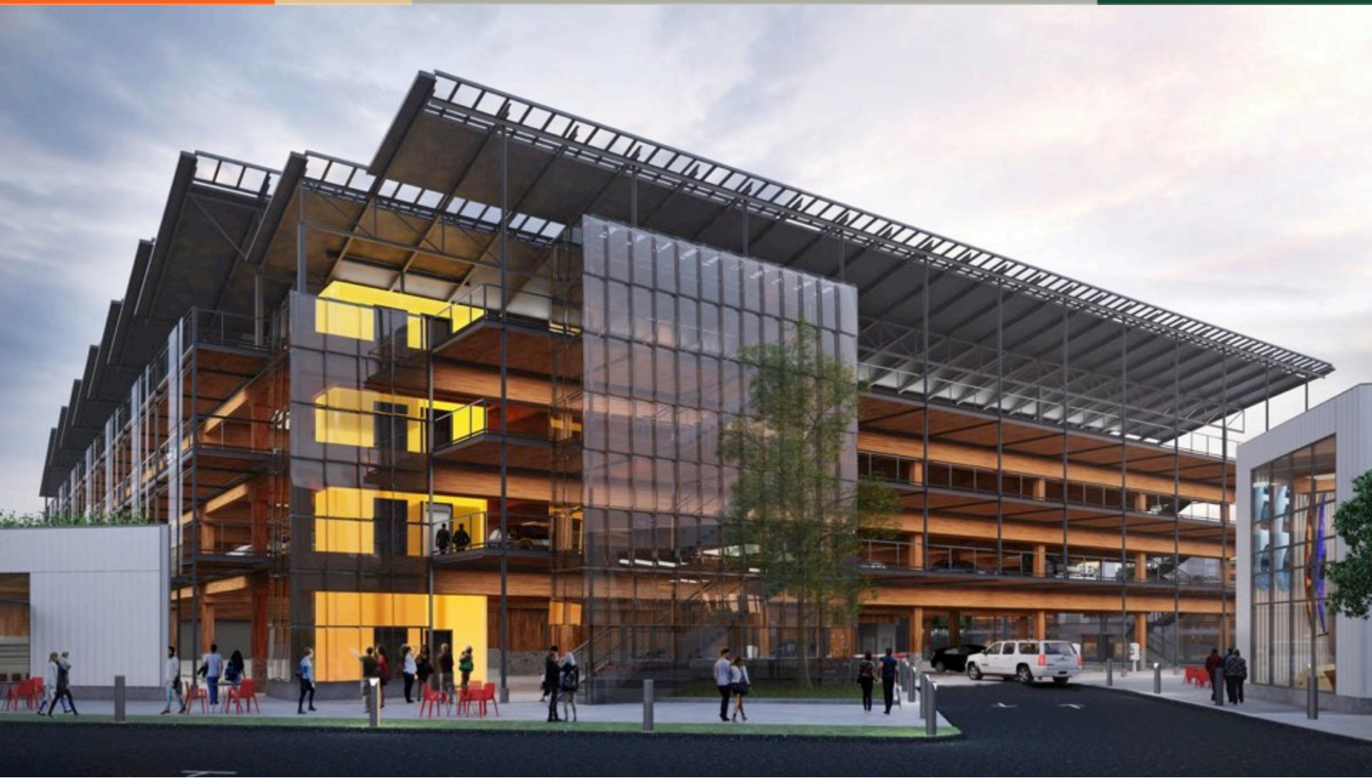
Glenwood Parking Garage, Springfield, OR SRG Partnership, 2018-19
