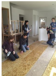
Students working on interior finishes
