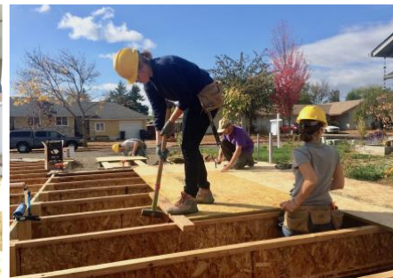
Students working on subfloor sheathing for house #5
