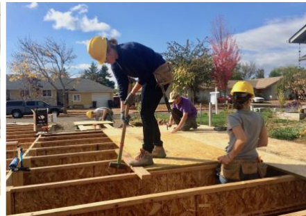
Students working on subfloor sheathing for house #5
