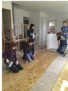
Students working on interior finishes
