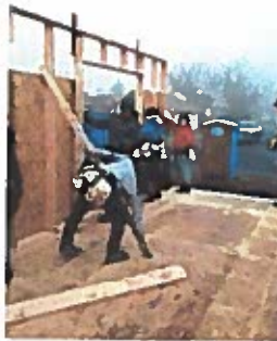
UO and LCC students building the frame during W14 term. The basic shell was erected in 4 weeks with the aid of a professional framer.
