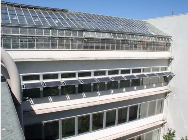
Fig. 1: Solar awning on the third floor of Pacific Hall. The modules are separated into two strings of six to minimize the shading problem on the whole system. The hallway on the second floor will be used as a control.
