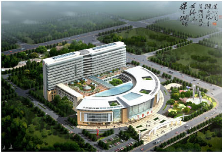
Completed project of scheme, preliminary design periods: Fuqing Hospital, Fujian Province, China ▲
