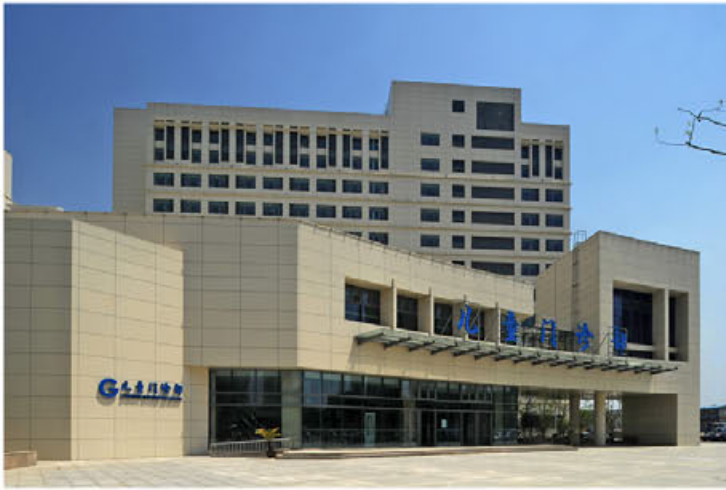
Completed project of whole design periods: ▲ Phase 2, Medical Center of Wuxi, Jiangsu Province, China
