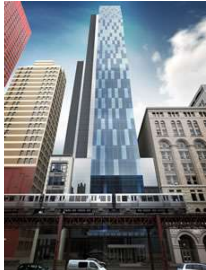
RU's Wabash Building, which will be Chicago's first LEED-certified skyscraper (expected completion 2012)
