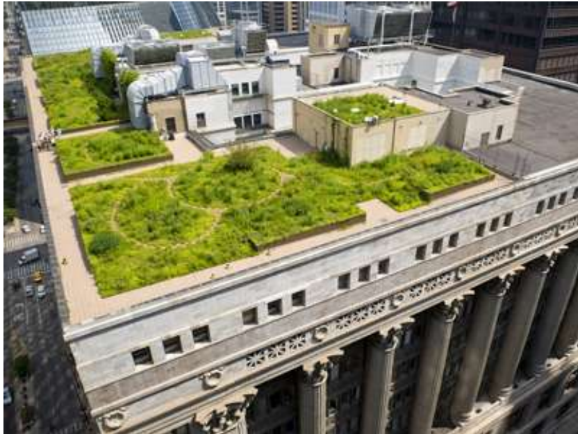
The green roof of Chicago's City Hall (source: City of Chicago)
