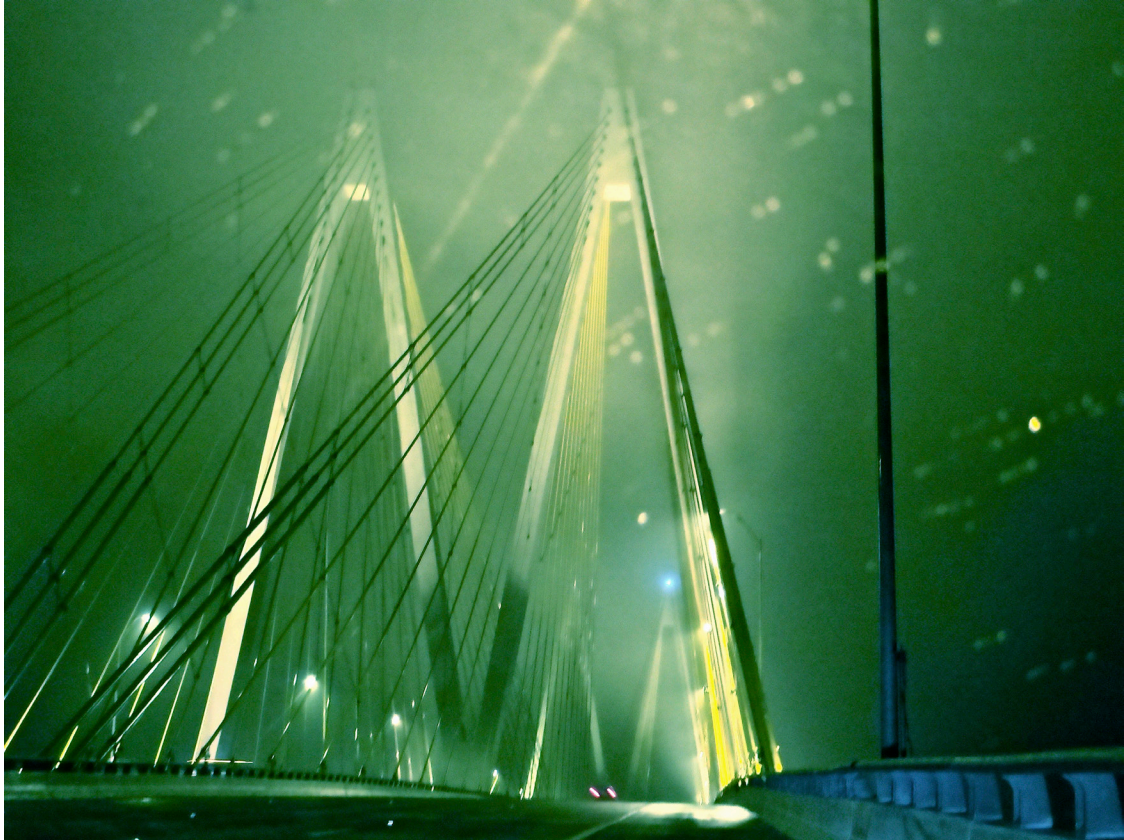
Fred Hartman Bridge Daniela Alarcon
