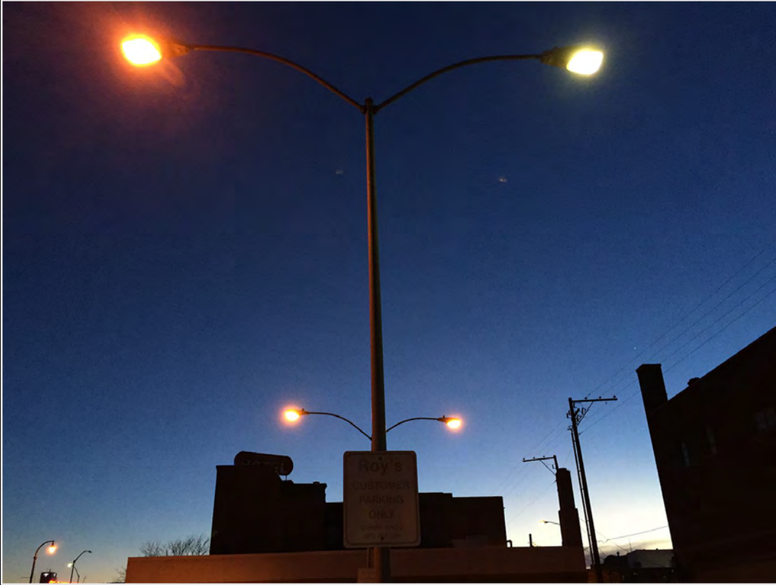
Sodium and Mercury Vapor Street lamps
