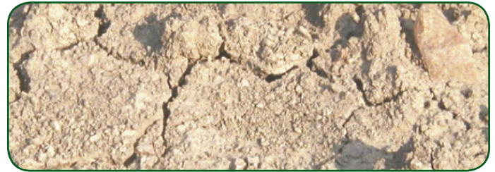
FIGURE 2. Surface crusting in mid-spring as a result of poor aggregation.
