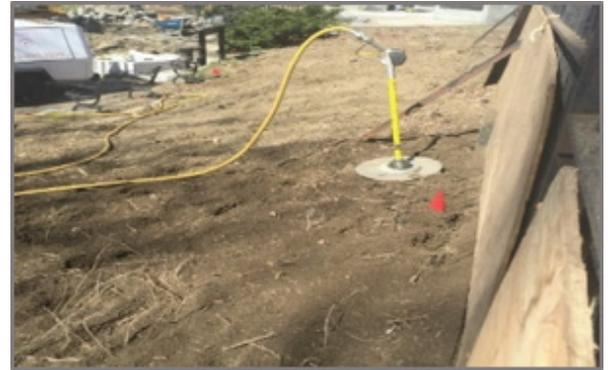
**Fig.4.** Air spade used to aerate and break up soil at Winthrop Square Park.
