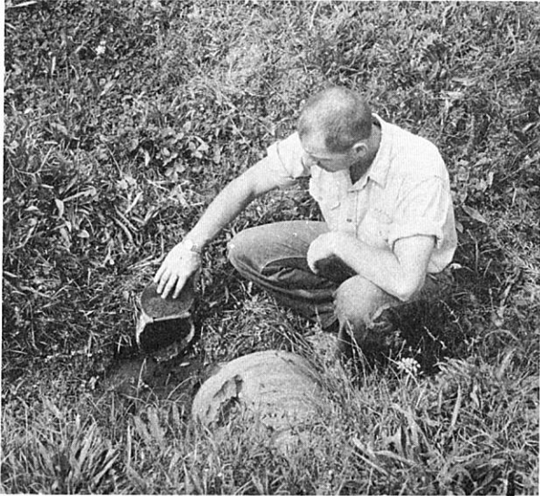
A flap gate rodent guard on an outlet pipe (P-529-5)
