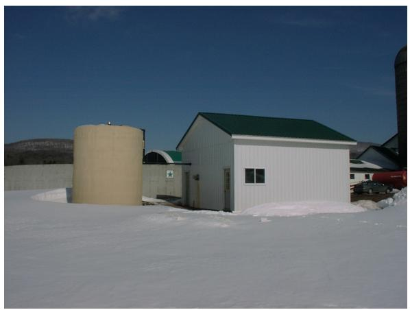
Figure 2. Vertical digester vessel and biogas utilization building on a 100-cow tiestall farm in NYS.
